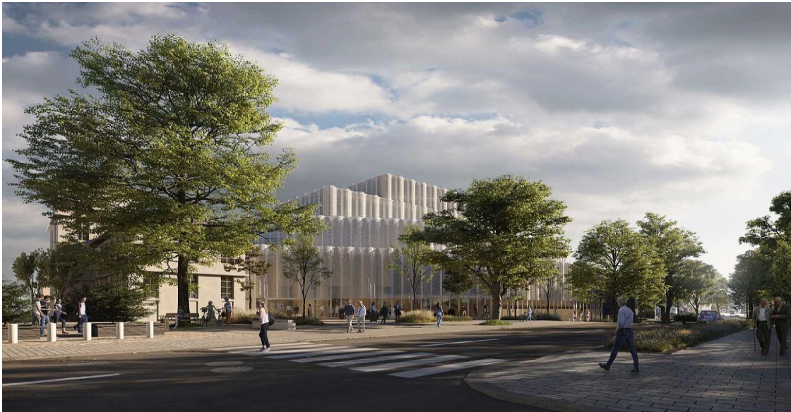
Figura 9. Kristiansund opera and culture house. Autoría de la revista An International Architecture Competition (Terry Pawsaon, 2010)
