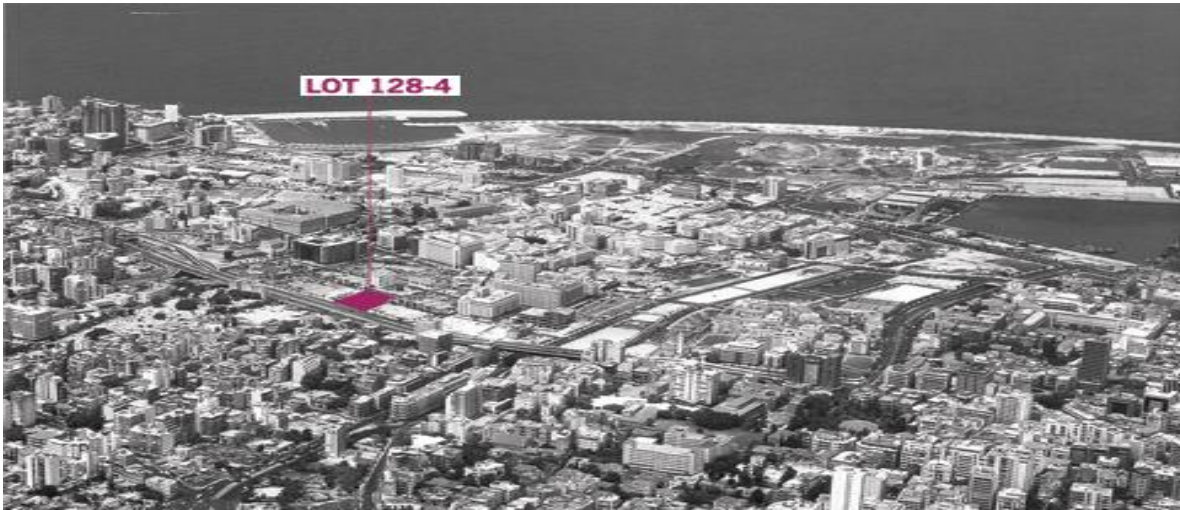
Figura 7. House of Arts. And Culture Project. Autoría de la revista An International Architecture Competition (Sánchez , 2009)
