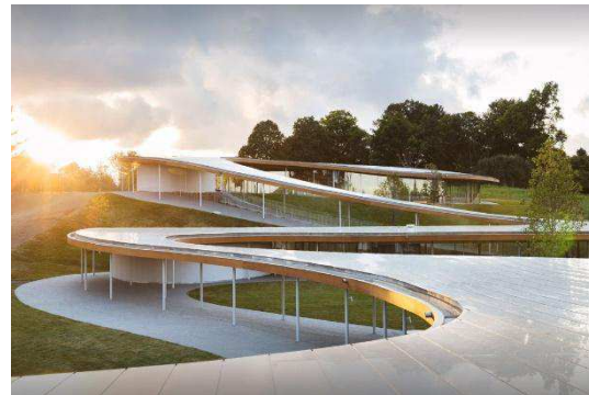
Figura 6 Grace Farms de SANAA https://www.archdaily.co/co/775407/grace-farms-sanaa
